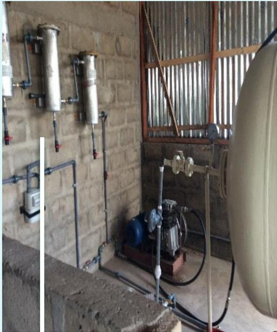
**Biogas Processing & Flow Controls**
