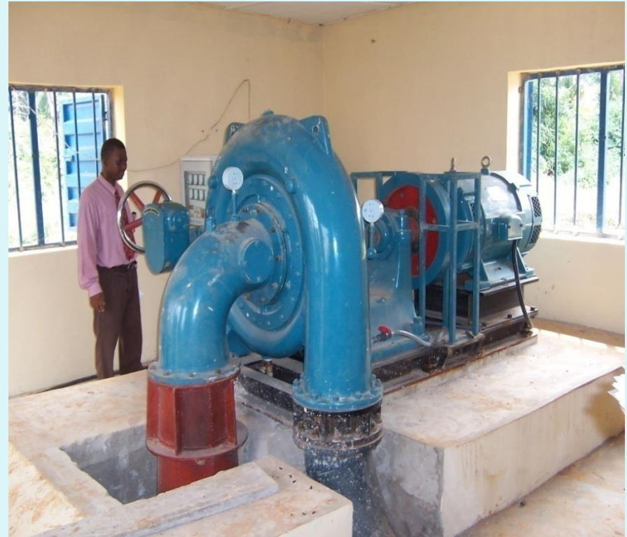
Penstock bifurcation into the 150 kW power house at Waya Dam, Bauchi State
