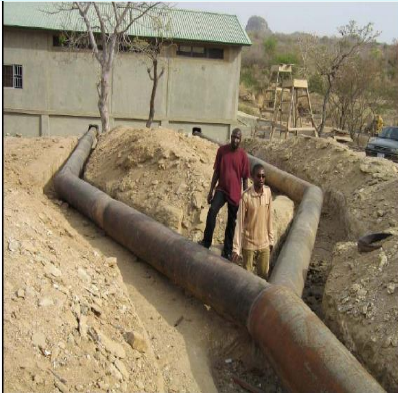
Penstock bifurcation into the 150 kW power house at Waya Dam, Bauchi State
