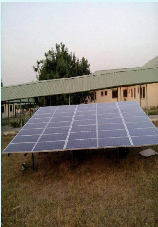
3kW solar PV mimi-grid in Talasse General Hospital, Balanga LGA, Gombe State (2013)
