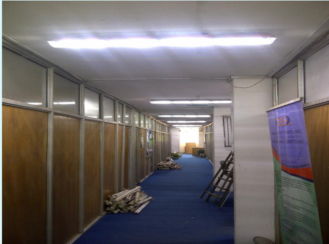
Retrofitting ECN Building with LED Lamps to half the lighting load of the building (UNDP-GEF Energy Efficiency project)
