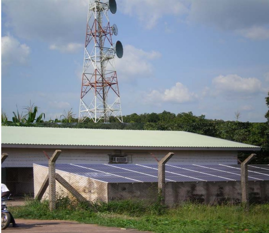
Solar PV for Telecommunication 20km Kaduna-Abuja Road, Nigeria
