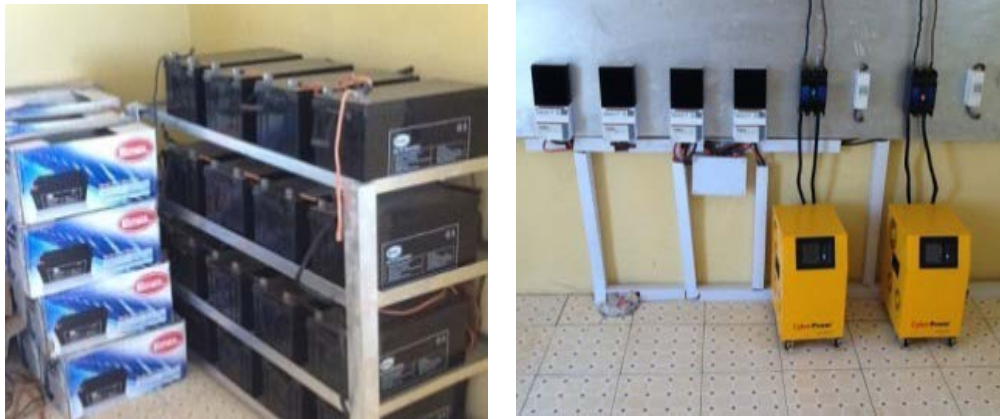
Battery Bank, Charge Controllers and Inverters in Control Room
